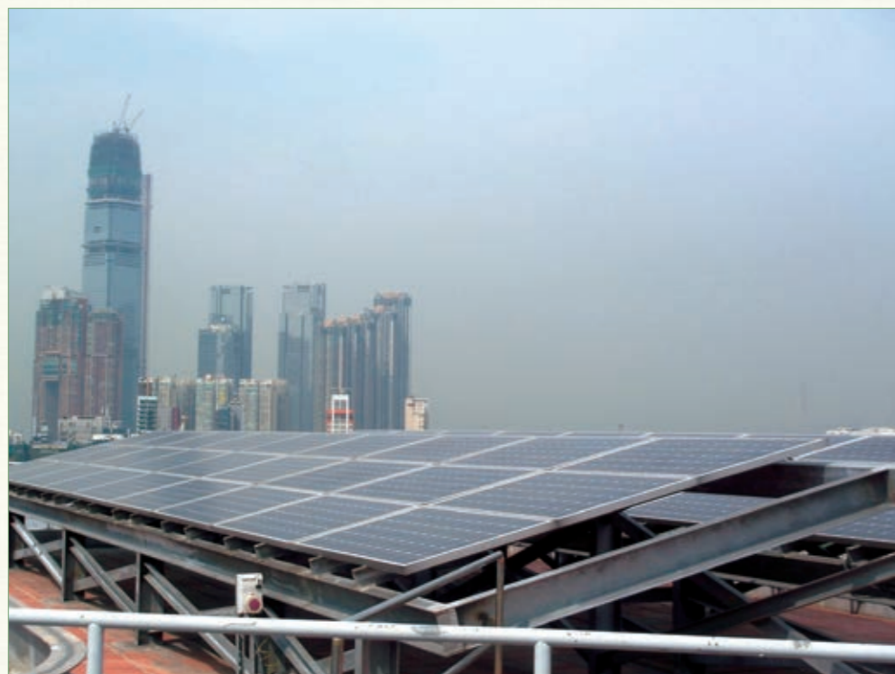
The Solar Photovoltaic System Installed on Roof 屋頂太陽能光伏板系統
