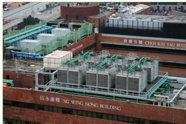
Water-cooled Chillers for Buildings on Campus 校園內樓宇的水冷式冷凍機
